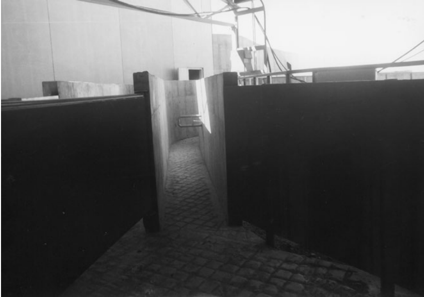
Fig. 3.9. Animals will tend to move from this darker forcing pen into a more brightly illuminated race, but they may balk at the sharply contrasting bright patch of sunlight on the inside of the race.
